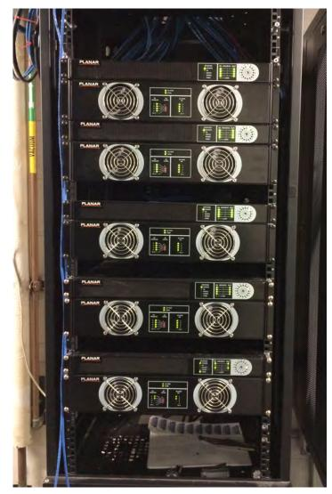
Planar Quad power and controller: 5 pairs of boxes (old Gen1 model, controller + power): 1 rack is enough for our 18 screens.
